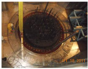
New Sandbox Cover Plates provided a waterproof seal that could withstand impact and support the weight of large components during the numerous cavity activities.
