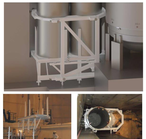
Because of logistics and limited space in the pool, the GTCC liners were to be located in the transfer canal. The addition of a separate frame to act as a seismic restraint was added after stand fabrication. Placement of the stand and frame into the final location required clearances of less than 1-inch (25mm) in some areas.
